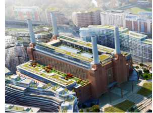
BATTERSEA POWER STATION PCE/MACE
